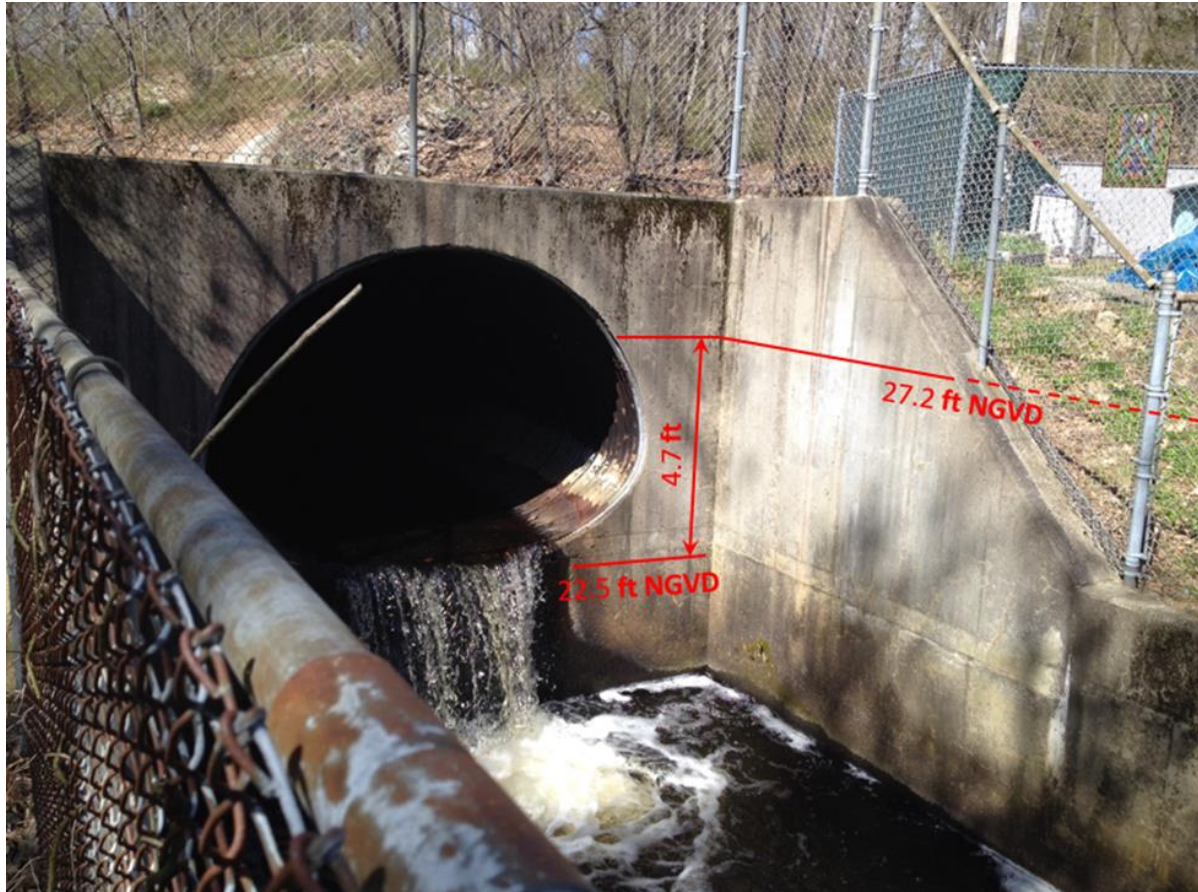
Figure 8-3: Expected Water Level in the Stilling Basin Under Alternative 2, with a Flow of 600 cfs.
