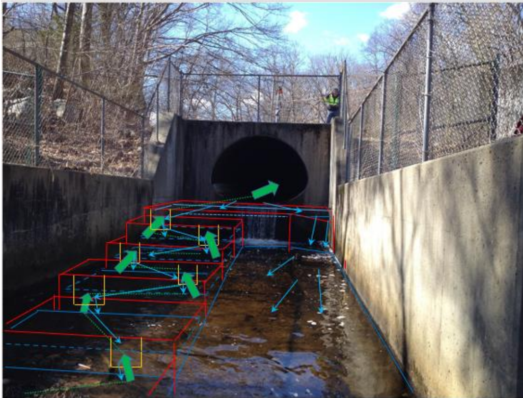
Figure 9-1: Alternative 2 - Fish Ladder on One Side of Stilling Basin, conceptual rendering. Fish passage illustrated in green, streamflow in blue.
